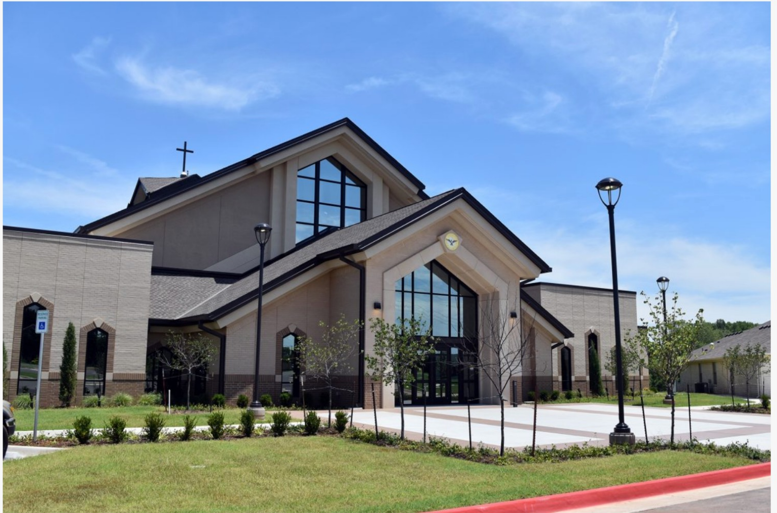
Mustang's Holy Spirit Catholic Church's new recovery was a project literally more than three decades in the making, completed in recent months. (Staff photo by Traci Chapman)
